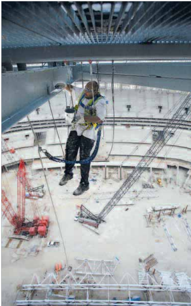
ABOVE LEFT: Nearly 300 feet above the stadium's playing surface, Chris Villanueva paints under the south arch truss.
